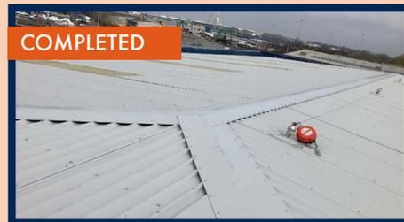
The pitched metal roof surfaces of this industrial building required thorough cleaning under high pressure to remove the build up of dirt that had accumulated on the roof over many years, this was particularly bad as a result of the exposed coastal location of the site. In addition the PVC Leathergrain Plastisol protective coating had been effected by primer damage causing almost total delamination.
