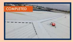
The pitched metal roof surfaces of this industrial building required thorough cleaning under high pressure to remove the build up of dirt that had accumulated on the roof over many years, this was particularly bad as a result of the exposed coastal location of the site. In addition the PVC Leathergrain Plastisol protective coating had been effected by primer damage causing almost total delamination.
